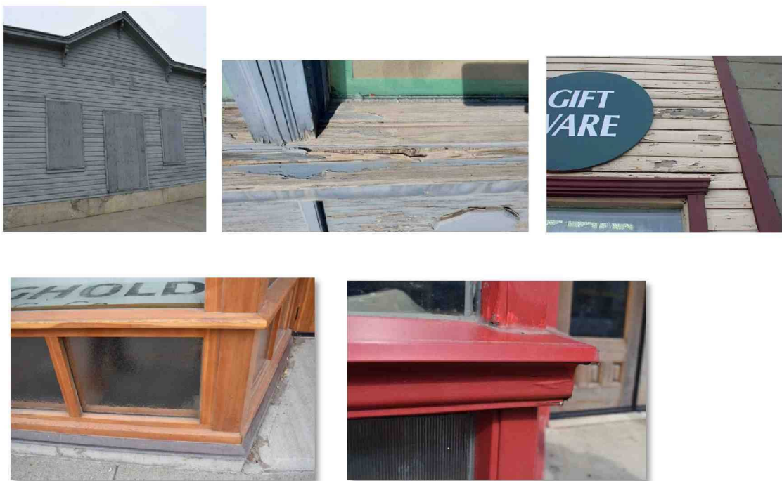
Figure 28: RT Barker and Renwick Building (2023): Bulkhead exterior woodwork should be retained and repainted with the appropriate paints (linseed oil) to conserve it for longer periods of time and as can be seen on the Renwick Building; cladding of wood components is generally avoided but may be necessary and appropriate in certain cases.
