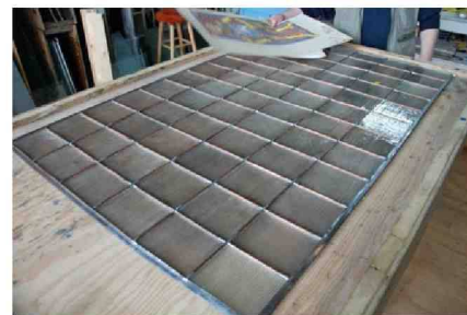
Figure 32: Great West and Renwick Buildings (2023) and Renwick Building Restoration (2010, 2014): As prism glass is no longer manufactured, conserve existing glass components through cleaning and repair.
