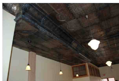
Figure 30: Grier Building pressed metal ceilings - exterior (2023) and interior (2019); Union Bank and Grier Block (2023) upper façade and roof pressed metal; Retain and maintain original historic pressed metal.
