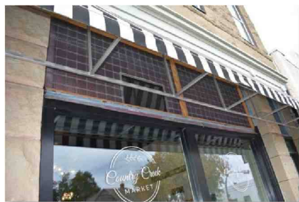
Figure 32: Great West and Renwick Buildings (2023) and Renwick Building Restoration (2010, 2014): As prism glass is no longer manufactured, conserve existing glass components through cleaning and repair.
