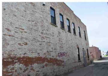
Figure 34: Grier Building (2023): Do not paint any masonry materials. If they have been painted, appropriately remove the paint as a part of a conservation plan to rehabilitate the masonry be it needed repair, repointing, fixing cracks, efflorescence, or spalling paint.
