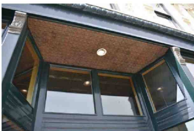
Figure 30: Grier Building pressed metal ceilings - exterior (2023) and interior (2019); Union Bank and Grier Block (2023) upper façade and roof pressed metal; Retain and maintain original historic pressed metal.
