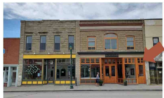
Figure 16: Reach Block, 1900s, 1973 and 202 photographs: Transom Restoration back to its original storefront design and material per historic photograph evidence; Restoration should seek to uncover the original materials and design of transoms and storefront features and avoid other architectural styles such as the mid-century one what was done on the upper photograph and remains on the Sam Chow Block to the right of the Reach Block.
