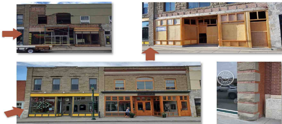
Figure 20: Reach Block, 2014, 2018, and 2020: Piers are a key structural and visual element of a historic building's façade design and should remain exposed and not covered up. Where they have been covered, they should be Rehabilitated or Restored so the original material is again exposed; the last photograph illustrates the Rehabilitated bottom of the pier on the McNeill-Mathews Block (2023).
