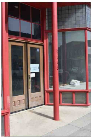
Figure 29: Renwick Building and Union Bank (2023): Historically used cast iron for structural columns and architectural decoration. Watch for corrosion on cast iron character-defining elements on a building.
