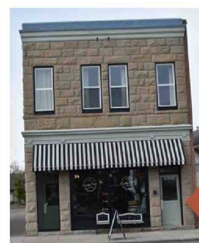
Figure 18: Great West Block (1920): Narrow recessed end façade entrances should be Restored or Rehabilitated even if a narrow recess access to the storefront and/or as access to the upper floor with an internal staircase. Work with the Town's Safety Codes resource and/or barrier free access to retain the original recessed entrance and seek alternative options to meet updated codes and provide for barrier free access.
