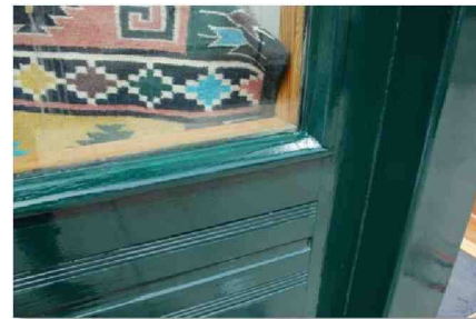
Figure 35: Renwick Building (2022) and Grier Building (2010): Identify the issues with peeling paint and repaint with a paint that will adhere and be long lasting with the material being painted.
