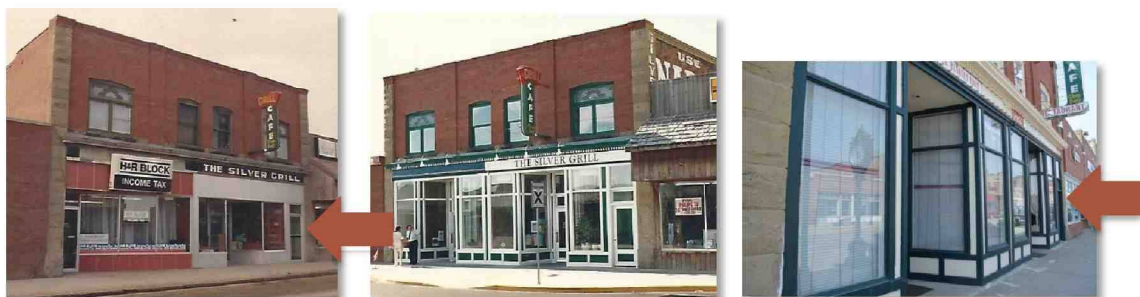
Figure 17: Leather Block (Silver Grill), 1983 display windows that were later rehabilitated back (1992) to an original display window pattern and type of the period of significance.
