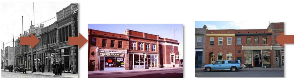
Figure 14: A. Y. Drug Store (early 1900s): Upper windows in the 1980s and 2016. Alterations and rehabilitation of upper windows must retain their original pattern and type including original material if possible (i.e wood double or single-hung with pane arrangement)
