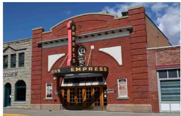
Figure 13: Empress Theatre, 1981 and 2022 photographs: The brick parapet and cornice were painted over, the paint later removed, and the parapet and cornice taken back to its original natural material including the parapet cap.
