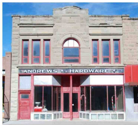
Figure 15: Renwick Building: Bulkhead Rehabilitation to original character-defining elements design however, metal clad over wood components is generally avoided but may be necessary and appropriate in certain cases..
