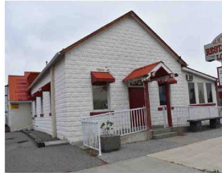
Figure 27: RT Barker (2008) and Legion Building (2023): Monitor, reporting stone masonry and do not paint masonry buildings as was done on the Legion's cast stone as it immediately ruins the integrity of the material and will spall as can be seen above the canopy.
