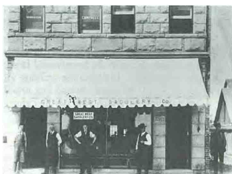
Figure 18: Great West Block (1920): Narrow recessed end façade entrances should be Restored or Rehabilitated even if a narrow recess access to the storefront and/or as access to the upper floor with an internal staircase. Work with the Town's Safety Codes resource and/or barrier free access to retain the original recessed entrance and seek alternative options to meet updated codes and provide for barrier free access.
