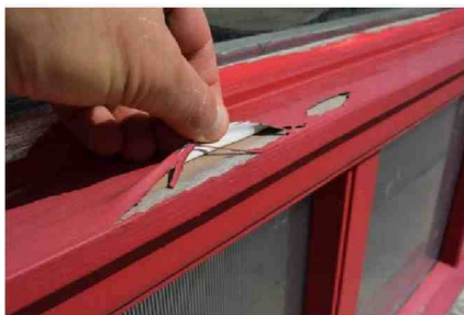
Figure 35: Renwick Building (2022) and Grier Building (2010): Identify the issues with peeling paint and repaint with a paint that will adhere and be long lasting with the material being painted.
