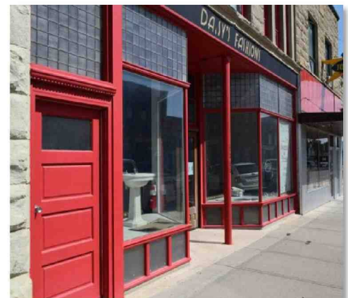
Figure 15: Renwick Building: Bulkhead Rehabilitation to original character-defining elements design however, metal clad over wood components is generally avoided but may be necessary and appropriate in certain cases..
