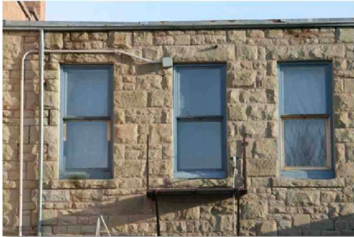
Figure 27: RT Barker (2008) and Legion Building (2023): Monitor, reporting stone masonry and do not paint masonry buildings as was done on the Legion's cast stone as it immediately ruins the integrity of the material and will spall as can be seen above the canopy.
