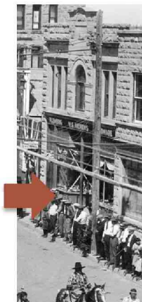
Figure 15: Renwick Building: Bulkhead Rehabilitation to original character-defining elements design however, metal clad over wood components is generally avoided but may be necessary and appropriate in certain cases..
