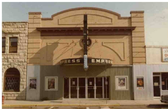
Figure 13: Empress Theatre, 1981 and 2022 photographs: The brick parapet and cornice were painted over, the paint later removed, and the parapet and cornice taken back to its original natural material including the parapet cap.
