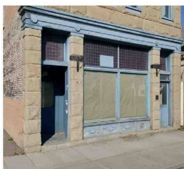
Figure 18: Great West Block (1920): Narrow recessed end façade entrances should be Restored or Rehabilitated even if a narrow recess access to the storefront and/or as access to the upper floor with an internal staircase. Work with the Town's Safety Codes resource and/or barrier free access to retain the original recessed entrance and seek alternative options to meet updated codes and provide for barrier free access.
