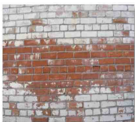
Figure 34: Grier Building (2023): Do not paint any masonry materials. If they have been painted, appropriately remove the paint as a part of a conservation plan to rehabilitate the masonry be it needed repair, repointing, fixing cracks, efflorescence, or spalling paint.
