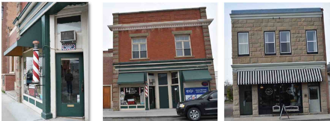
Figure 21: McNeill-Mathews Bloc and Great West Block (2023): Canopies and awnings were not prevalent in Fort Macleod historically however the McNeill Matthew Block has retained a canopy and the Great West Block historically added one back to the building façade which is appropriate to Restore per the guidelines.
