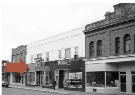
Figure 16: Reach Block, 1900s, 1973 and 202 photographs: Transom Restoration back to its original storefront design and material per historic photograph evidence; Restoration should seek to uncover the original materials and design of transoms and storefront features and avoid other architectural styles such as the mid-century one what was done on the upper photograph and remains on the Sam Chow Block to the right of the Reach Block.
