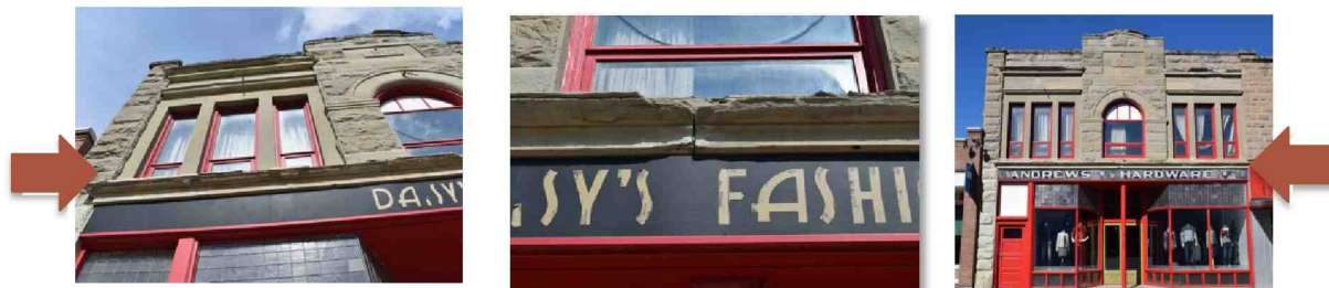
Figure 19: Renwick Building (2022): Lower cornices are often altered and/or deteriorate over the years as is happening on the Renwick Building. When Rehabilitated the lower cornice should only include rehabilitation or restoration of the original materials, design, and these components not altered.
