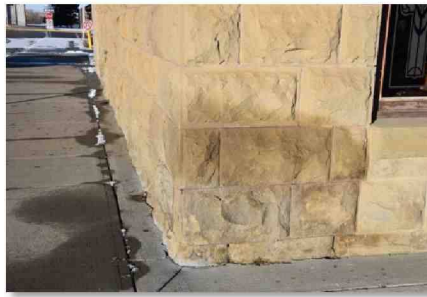
Figure 26: Bank of Commerce (2023) and Queen's Hotel (2015): Monitor, repair, and/or replace, stone masonry as needed using the guidelines for appropriate conservation intervention.
