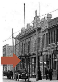
Figure 16: Reach Block, 1900s, 1973 and 202 photographs: Transom Restoration back to its original storefront design and material per historic photograph evidence; Restoration should seek to uncover the original materials and design of transoms and storefront features and avoid other architectural styles such as the mid-century one what was done on the upper photograph and remains on the Sam Chow Block to the right of the Reach Block.
